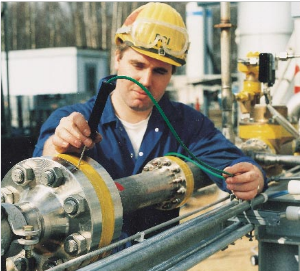
Carrying out a leakage test on a hydrogen system
